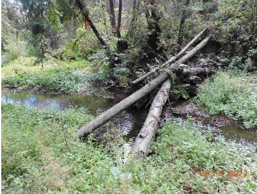
Photo 9. Partial log jam present in 2021 has been reduced, but the stream channel upstream (to the right) has been rearranged from the far bank to the near bank (foreground). The formerly deep pool (now under the logs) at the large redwood stump on the far bank is now half filled with sediment and is now largely isolated from the main current and stagnant; this has eliminated the fast-water feeding habitat and few fish were present. The stump pool does provide high flow over-wintering habitat.
