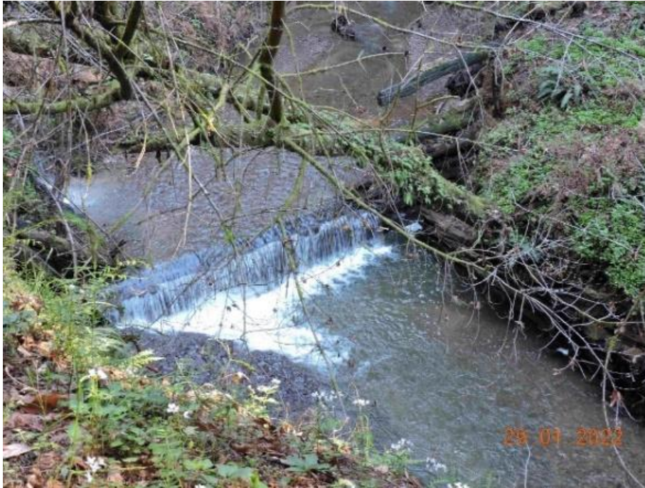
January Photo 44. About mile 4.0. Log weir with level gravel channel upstream. Three foot jump required from the partially filled pool.
