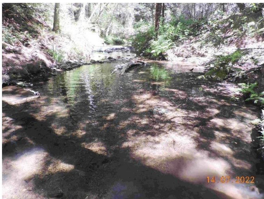
Photo 76. Mile 5.25, looking upstream. Fish sampling pool upstream of Humboldt crossing is now two-thirds filled with fines and gravel, eliminating undercuts on left bank.
