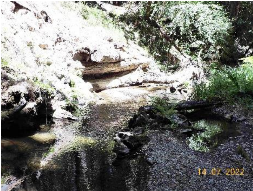
Photo 68. Mile 4.9. Upper fish sampling pool with San Mateo County stacked log bank protection upstream and stacked boulders and root wad bank protection downstream. The pool, one of three fish sampling habitats with significant filling in both 2021 and 2022, is now mostly filled, with undercut banks eliminated.
