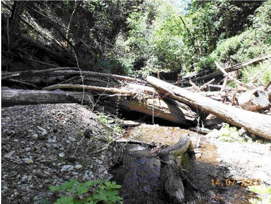
Photo 51. Mile 4.1+. View of jam from upstream. Jam is 5 ft high, 35 ft wide, and 35 ft long. Possible fish passage under the jam along the right bank. The well-anchored jam is a potential serious fish passage barrier that should be modified.
