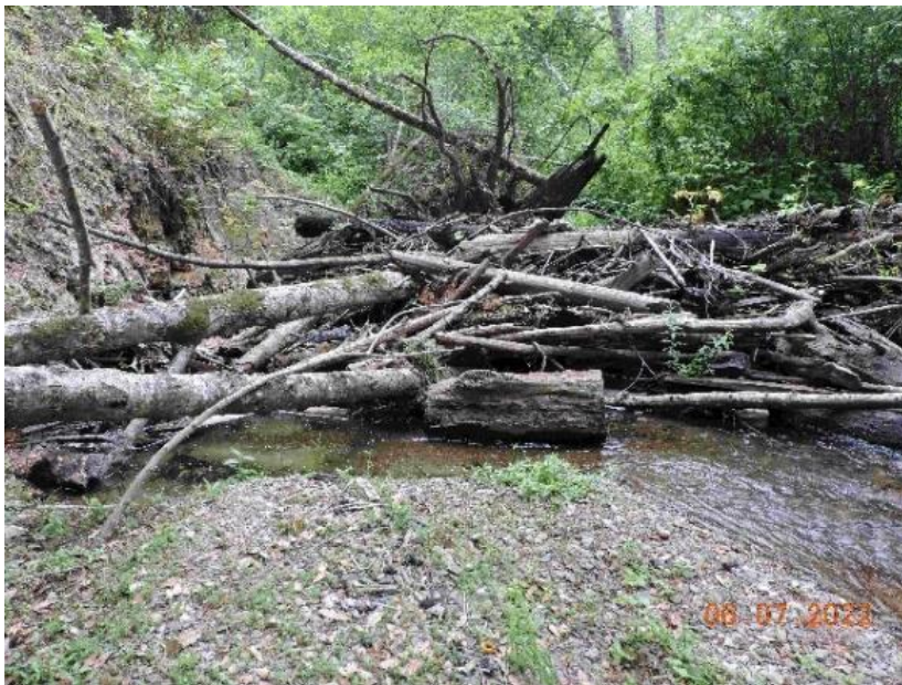
Photo 14. Mile 2.8, looking downstream. Preexisting logjam partially burned in 2020, but with added wood since. Possible fish passage underneath near left bank, but a potential fish passage problem; should be monitored and modified if needed. Backwater at the jam resulted in filling the upstream pool with sediment.
