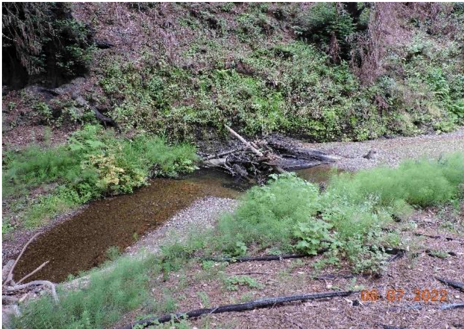
Photo 41. Mile 3.9. Leveled gravel channel, with filling of long, deep pool, except around the old large rootwad/log in center of pool (annual fish sampling pool). Entrenched channel with 10 ft high near-vertical right bank.
