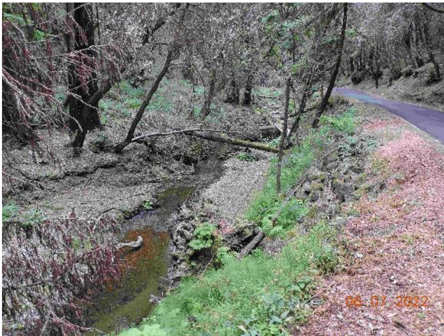
Photo 34. Mile 3.5. Shallow entrenched roadside channel, showing high flow scour line on left bank and San Mateo County stacked boulder bank protection on right bank. Level channel, despite some added wood.
