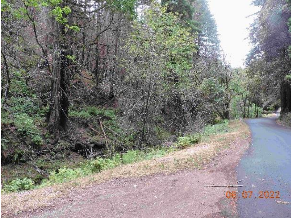
Photo 25. Mile 3.1, looking downstream from pullout. Road closely adjacent to shallow entrenched channel. Few right bank trees.
